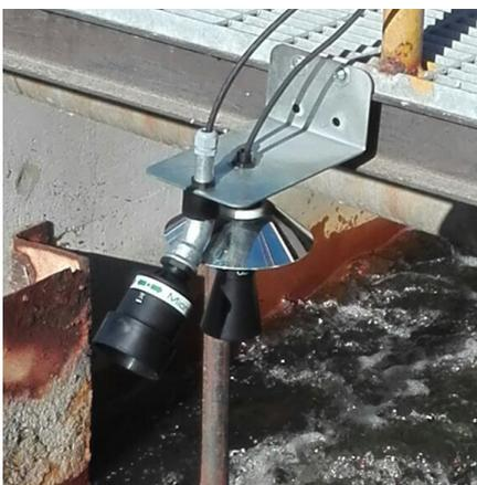
MicroFlow and dBMACH3 in a wastewater application
